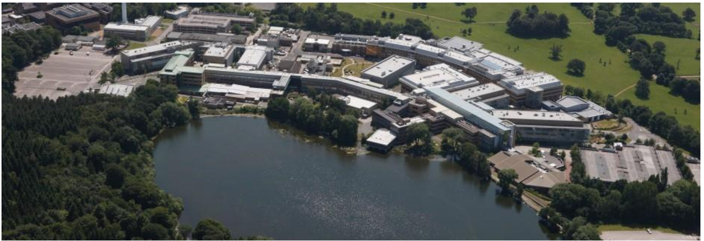
Aerial view of the Alderley Park site
