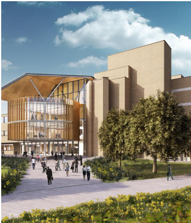
Alderley Park – Refurbished CTL building
